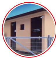
container stations and indoor switchgears
