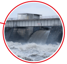
water and biogas plants bays
